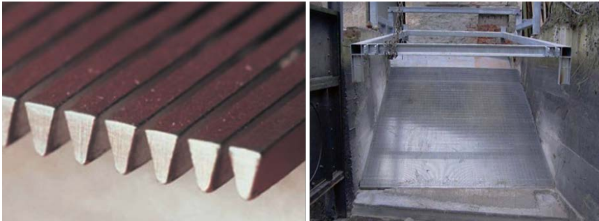
Abbildung 12: Wedge-wire screen (links: Dumont et al., 2005; rechts: Adam & Lehmann, 2011).
